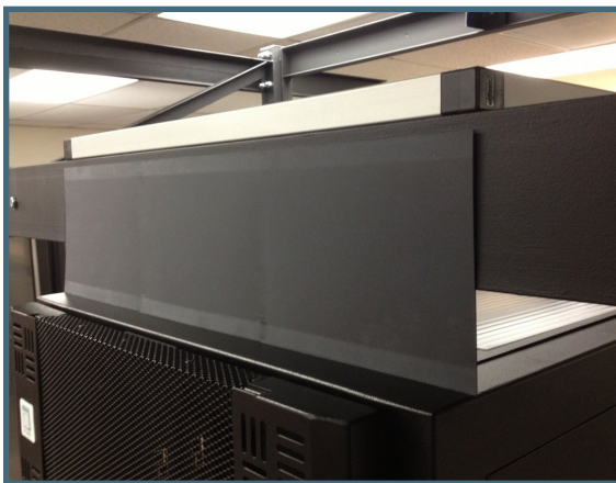
Fill Gaps Above Racks
